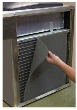
Figure 3-8 F122 Condenser Filter Removal
