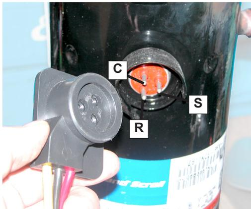
Figure 3-3 Compressor Connection
