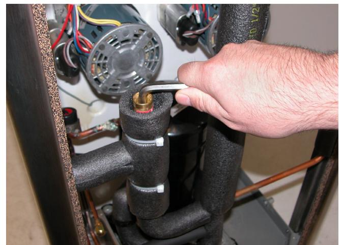
**Figure 3-8 Hot Gas Bypass Adjustment**
